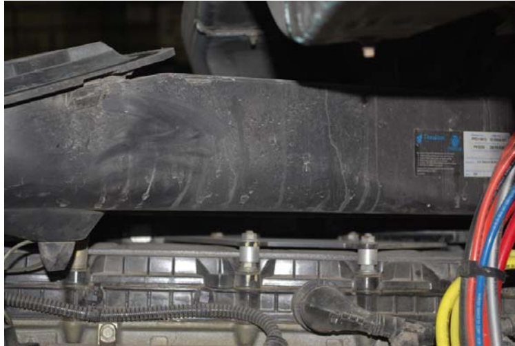
Figure 2 - Left Side Engine Air Filter Housing
