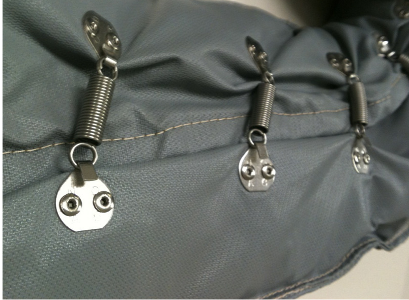
Figure 4: Insulated Blanket Installation
