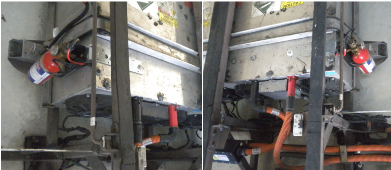
Fig 20 – Street Side and Curbside Complete
