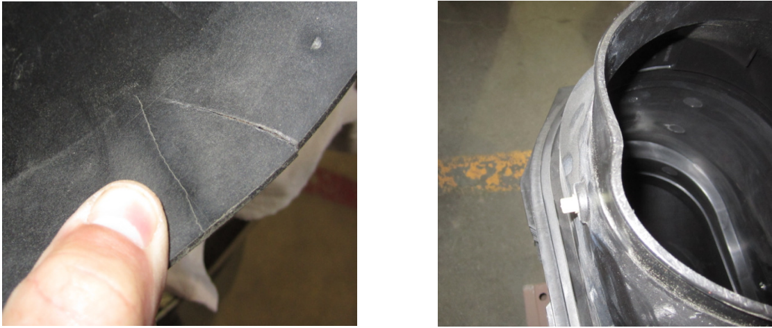
Figure 9: Air Filter Housing Inlet/Outlet Flange Damage
