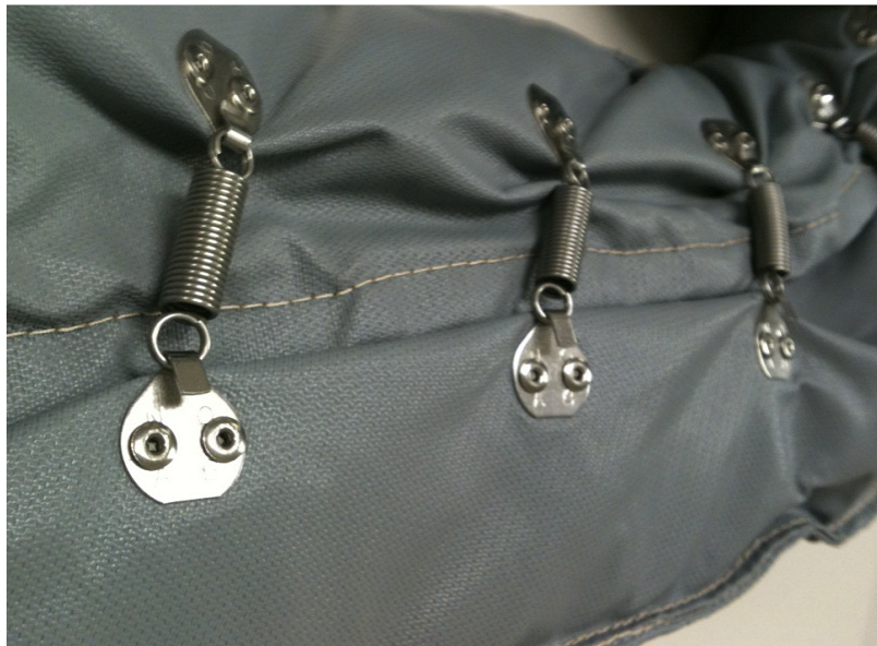
Figure 4: Insulated Blanket Installation
