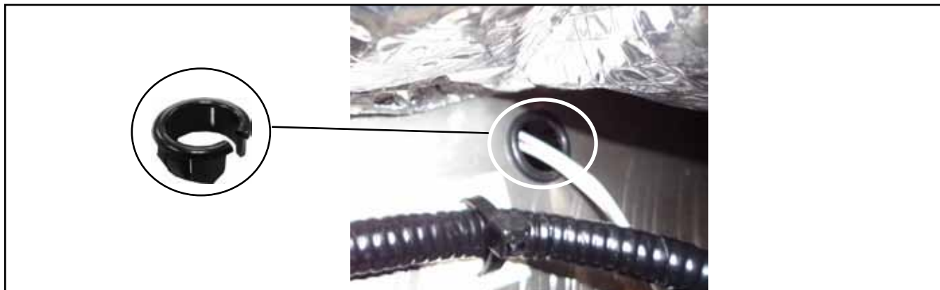
Figure 2 - Plastic Bushing Installation on the Structural Ceiling Beam
