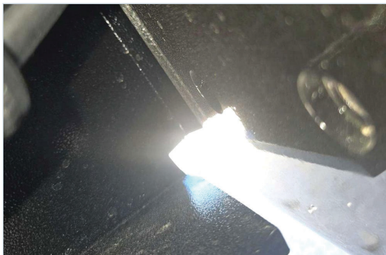
Fig. 1 — Reported failure. A complete break along the bend of the tongue. Daylight through the joint confirms the crack has gone through.
