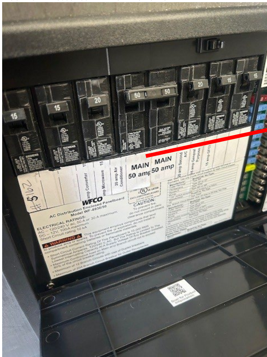
FIGURE 3 - WF-8930 - 50 AMP DISTRIBUTION CENTER
