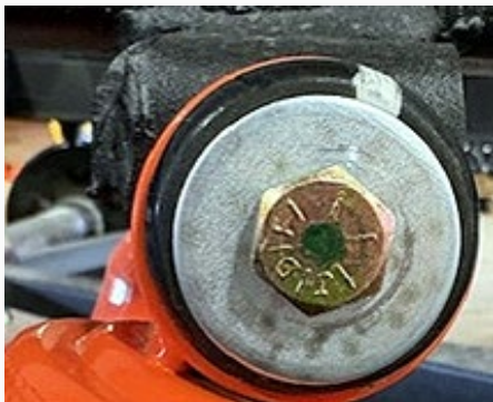
Exemplar — Completed installation with green epoxy paint marker on newly installed Grade 8 bolt.
