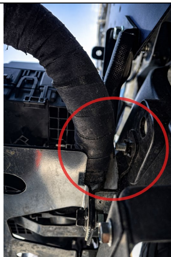
Step 7 – Inspection (refer to NOTE in service procedure)
