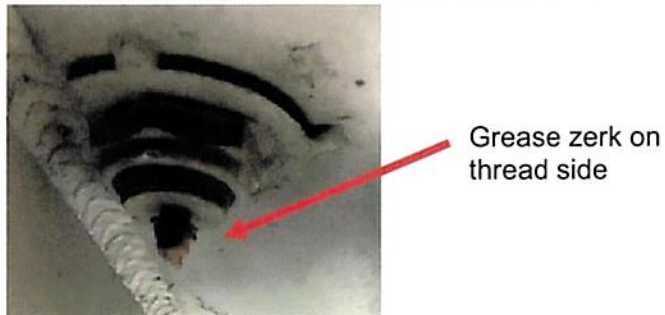
Grease zerk on thread side
