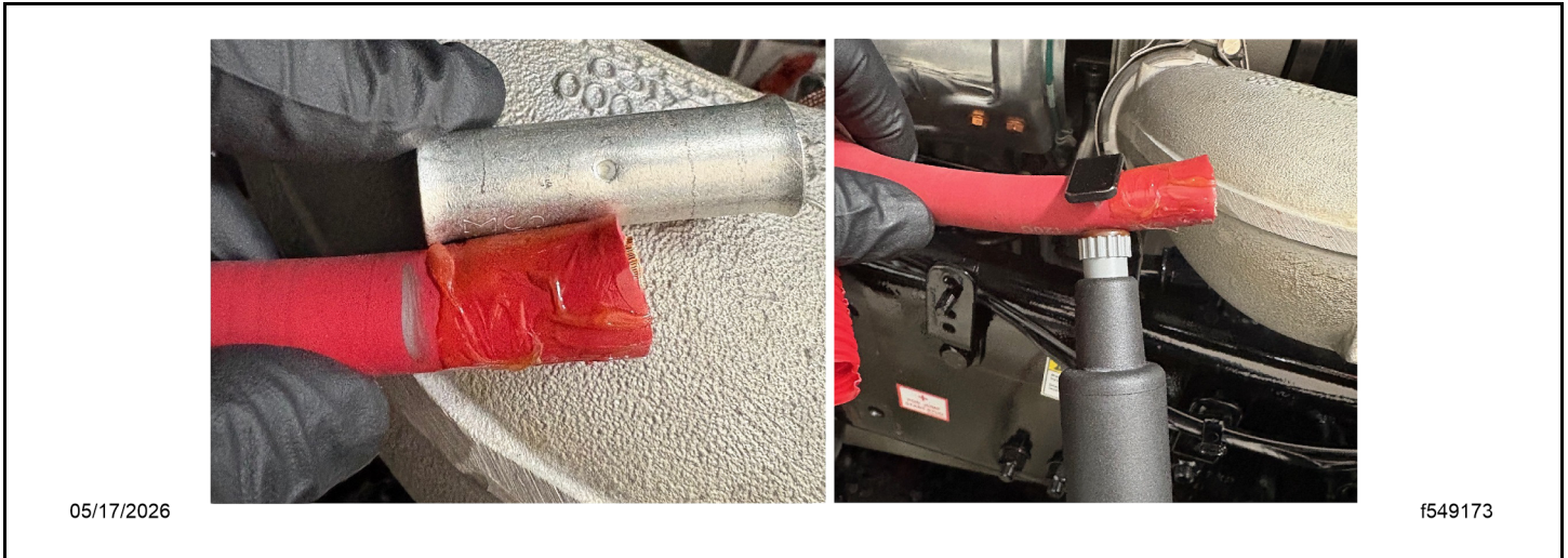
Fig 75, Removing the Insulation
