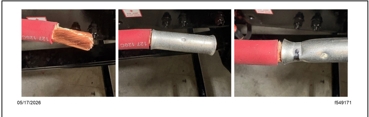
Fig 159, Installing and Crimping the Terminal
