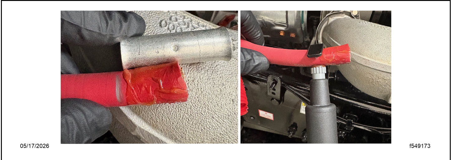
Fig 145, Removing the Insulation
