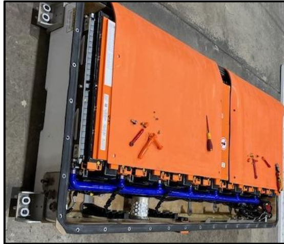
Figure 4: Terminal Covers Installed Back on Battery Modules
