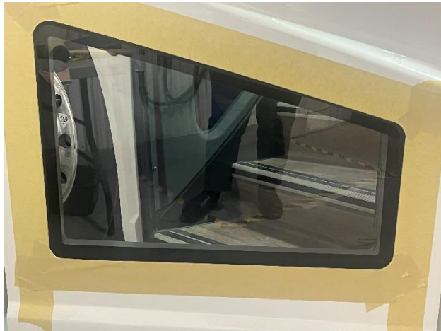
Figure 1: Outside Perimeter of Entrance Door Lower Window
