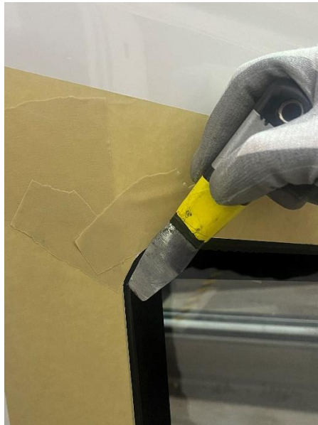
Figure 4: Removing Remaining Sika with Putty Knife
