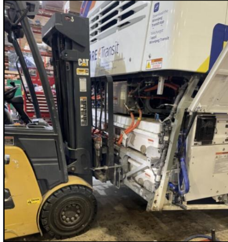
Figure 75: Rear Rack Assembly with ABS Packs Installation
