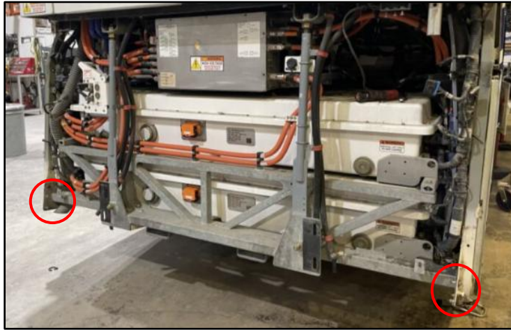
Figure 13: ESS Cradle Cross Member Hardware Removal
