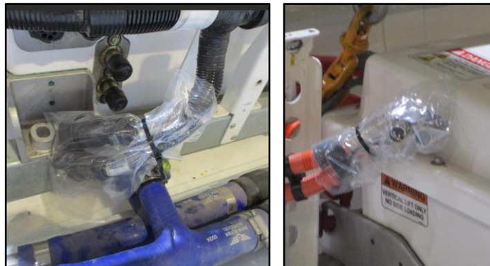
Figure 29a & 29b: Bagged Electrical Connectors
