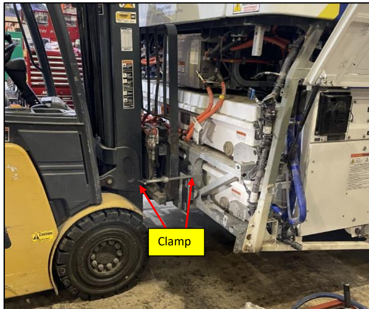
Figure 18: ESS Cradle Secured to Forklift
