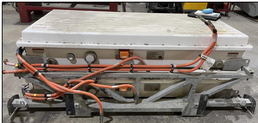
Figure 19: ESS Cradle on the Floor
