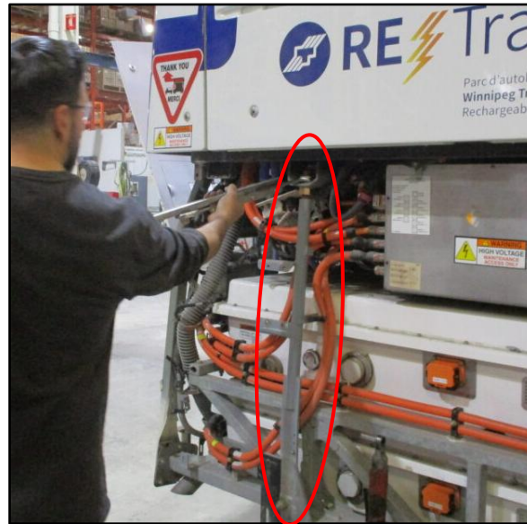
Figure 9: Loosening Strut Hardware
