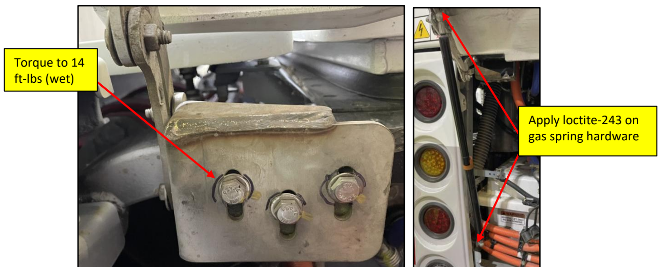
Figure 92a & 92b: ESS Door Reinstallation
