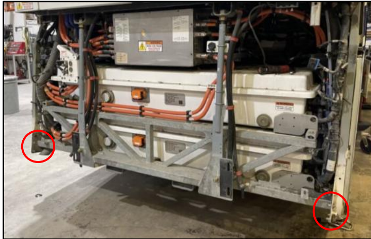
Figure 13: ESS Cradle Cross Member Hardware Removal
