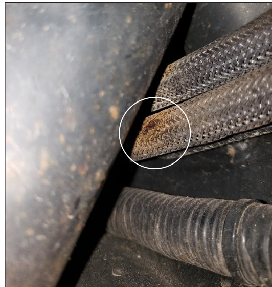
Figure 7 — Fuel Line Cosmetic Damage Example— Replacement Not Needed
