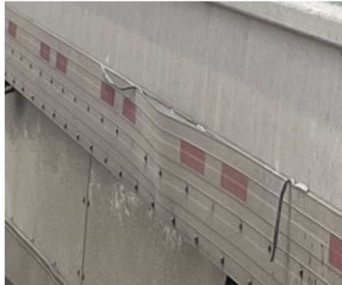
Figure 4: Baserail separation from sidewall.
