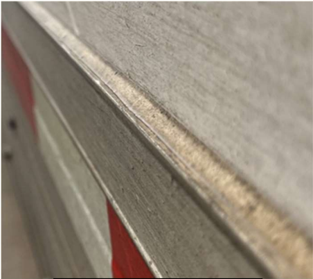
Figure 5: Caulk cracking.
