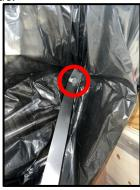
b. Place tape over the holes to ensure the bag is completely sealed.
