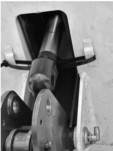
Figure 2 – Temporary support for cylinder rod end.
