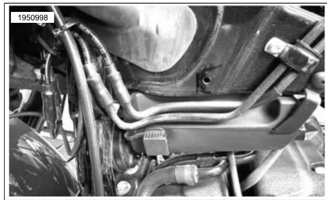
Figure 2. Inspection Area (Incorrect Brake Line Routing)
