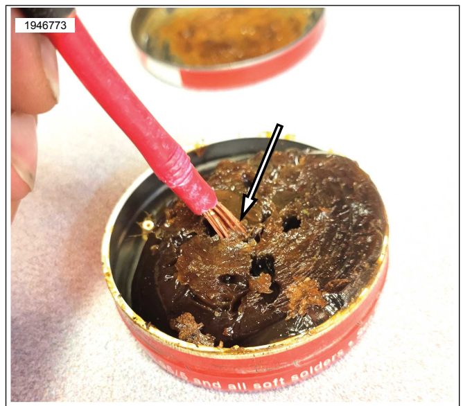
Figure 15. Prep 1: Apply Flux to Stripped Wire
