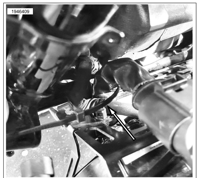
Figure 25. Loose Cable Strap
