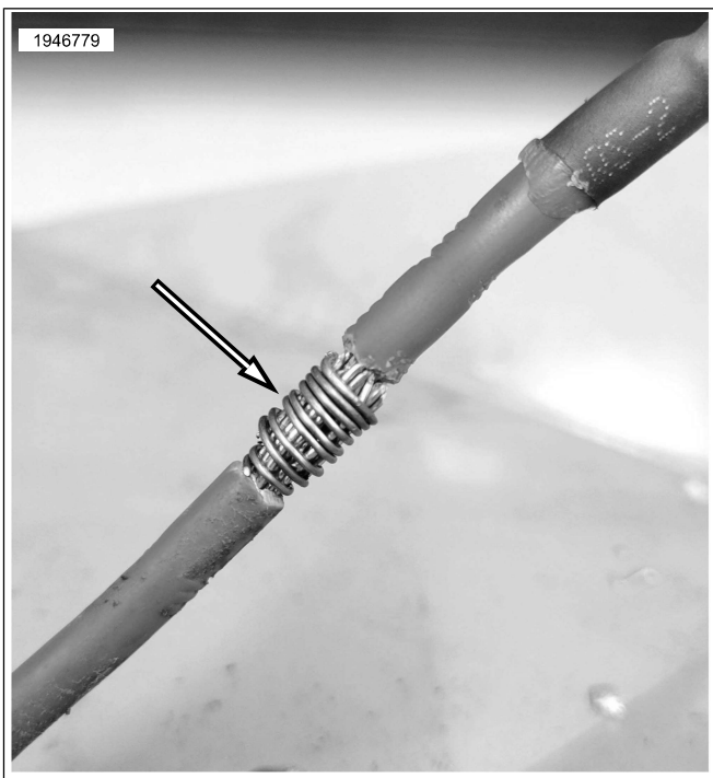
Figure 17. Prep 3: Wrap Joint with Thin Gauge Wire
