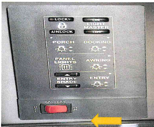
(2.1) Locate the Battery Disconnect at Entry door and turn off.
