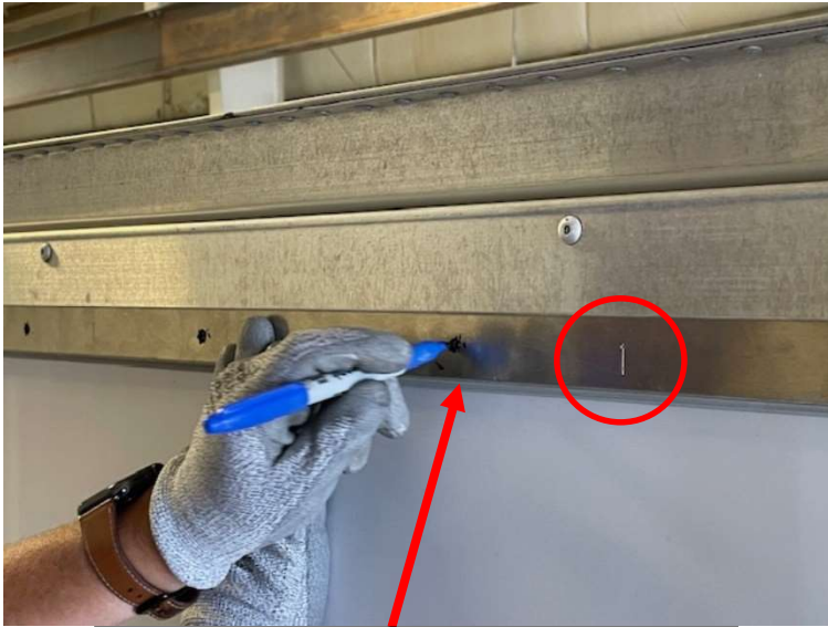
The edge of the Marking Guide should be lined up with the bottom edge of the Toprail.
