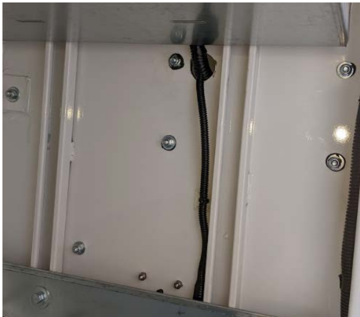
Image 4 - Roadside wire routing (new light box & license plate light)
