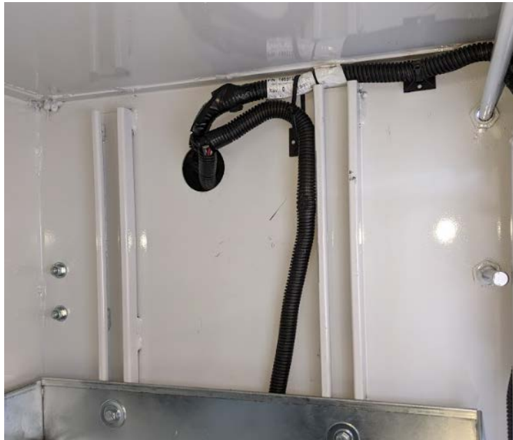
Image 3 – Roadside wire routing (upper light box)
