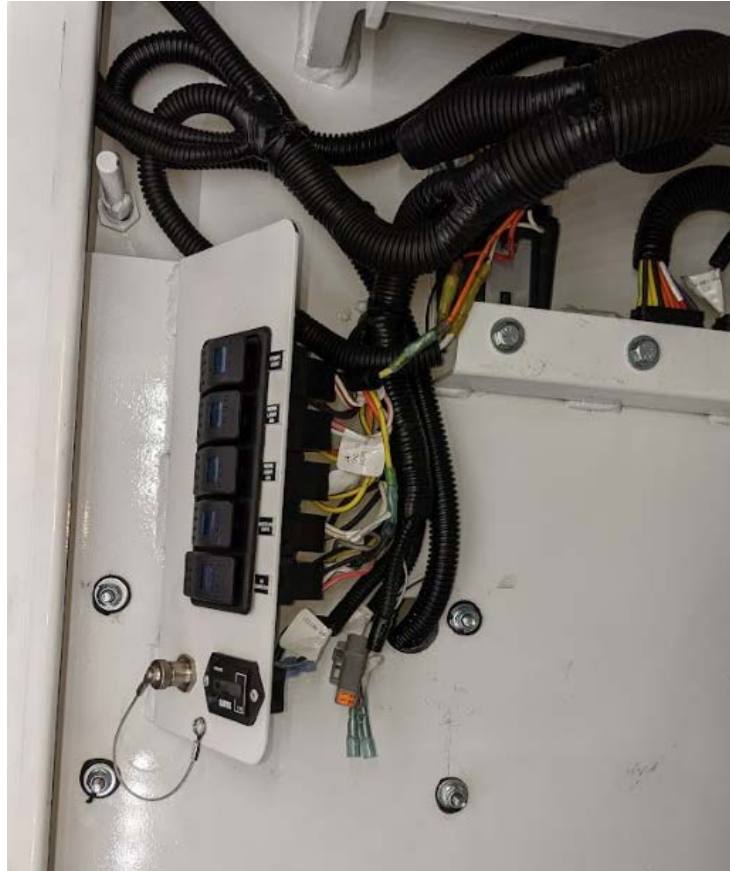
Image 5 – Curbside wire routing
