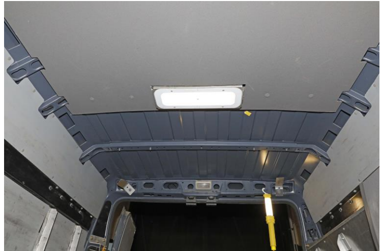
Figure 5 – Rear Ceiling Panels Removed
