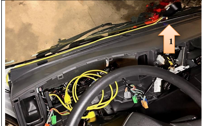
Figure 27 Current Cable Routing (painted yellow for reference.) 1. Tape Location
