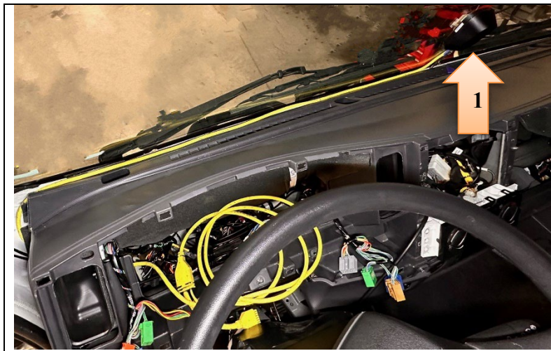
Figure 61 Current Cable Routing (painted yellow for example.) 1. Tape Location
