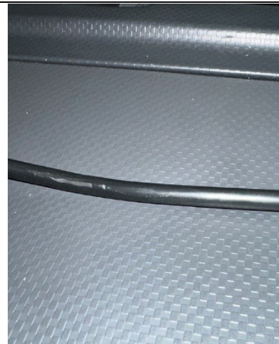
Figure 19 OK Harness: light scuffing or witness marks from handling with no major deformation of the insulation.
