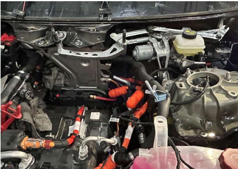
Figure 7, HV electrical connectors with protective covers (001 589 06 91 00)
