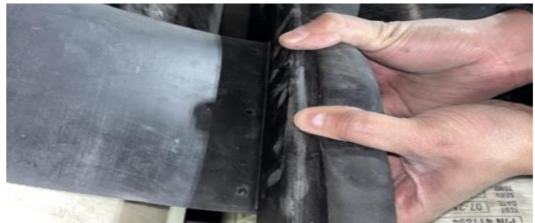
Figure 26 - Rubber kit being installed.
