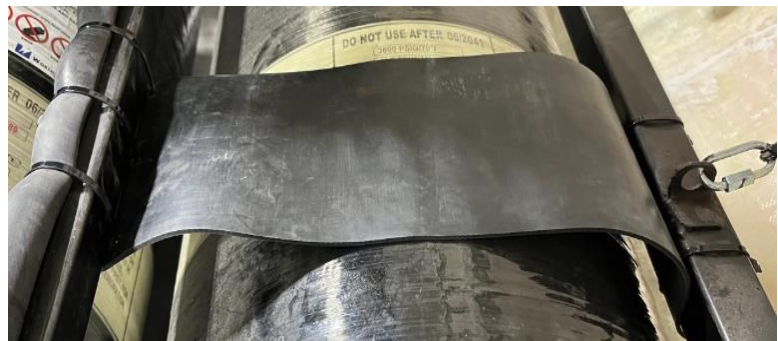
Figure 27 - Rubber kit installed.
