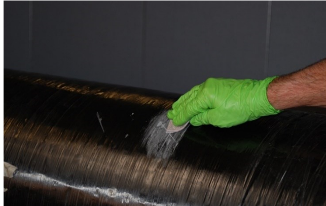
Figure 21 - Tank being sanded.
