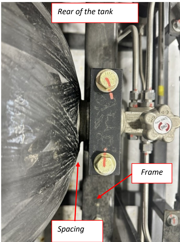
Figure 7 - Spacing between CNG tank and cradle(rear).
