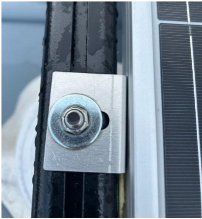
Figure 1C, updated stainless steel bracket, washer too large for nut.
