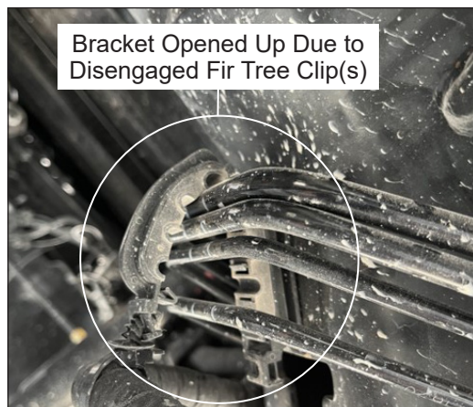
Figure 11 — Loose Plastic Fuel Line Bracket
