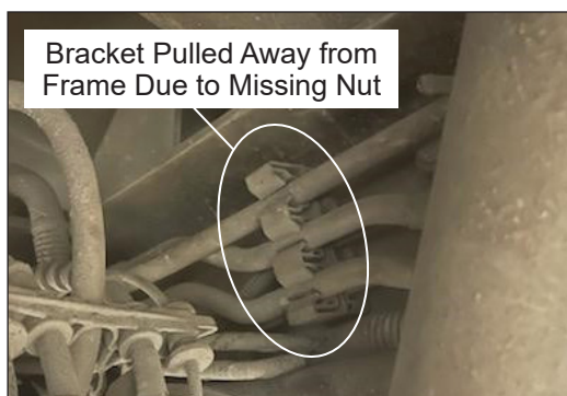
Figure 7 — Loose Plastic Fuel and Brake Line Bracket
