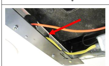
Verify the yellow 12/2 NMD wire is missing a grommet where it runs into the roof frame.
