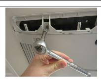
Remove the 6 hex drive screws from the diffuser housing.
