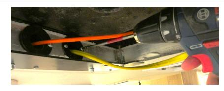
Secure grommet in place with the two self-tapping screws into the frame.
