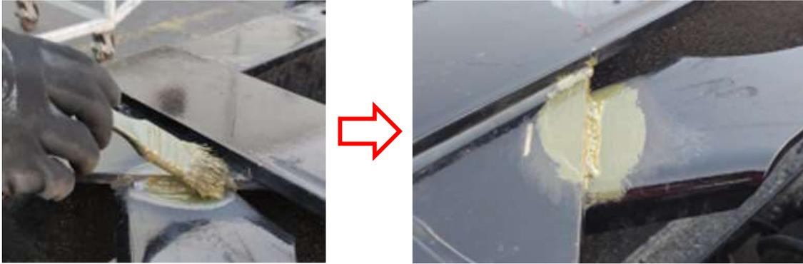
15. After primer is dry, apply paint over all areas repaired, on top and under diagonal brace.
