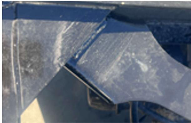
16. For those diagonal braces that have a missing/partial (less than 50%) welding , **it's not necessary** to apply welding underneath, bracket X520-DD018-H01 has to be installed (over the area already repaired) ONLY for those diagonals with missing/partial weld on bottom hole as shown on picture of step 3 & 4.
