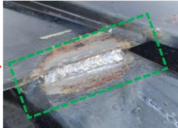
11. Using a chisel, remove weld spatters from weld, then use a carbon steel wire cup brush or a wire brush to clean better the welded area.
