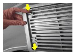
Push both clips down and reinstall the top clip screw of the vent. Start screw by hand into the metal bracket on the vent frame. Be careful not to strip the screw or overtighten and crack the plastic.
