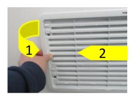
With both clips up, remove the vent by pulling on the left side of the vent and then sliding it out. Set vent aside.
