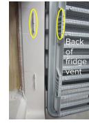
Reinstall vent by lining up the tabs on the right side of the frame with the slots in the grill and swivel the left side in.
