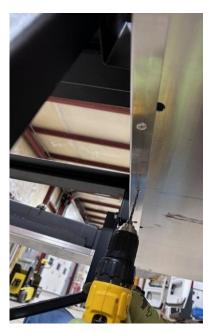
Place a spacer on each side of the L-channel that secures the underbelly to the fame. This will allow the bracket to sit flat against the frame. Attach the spacers using a 12" strip of VHB tape.
