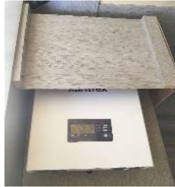
(FIG 2 – 1 OF 2) POWER INVERTER CABINET
