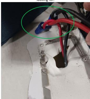
4. The wire nuts shown in the above image will need removed and replaced with new butt connectors. Be careful to reconnect the wires exactly as they were connected (+positive to +positive and -negative to -negative).
