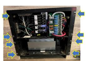
Line the two tabs up at the bottom of the cover to align it with the power center.
