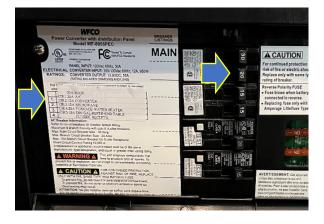
Remove the two screws securing the cover.
