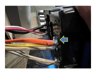
Pull the Romex wire for the A/C out of the power center and tape the end of the wires. Coil the wire up behind the power center.
