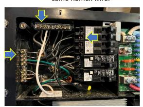
On the back of the power center, loosen the wire clamp to the Romex wire for the A/C.
