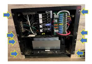
Using a #2 square bit screw driver, loosen the screw and remove the black wire for the A/C breaker. Trace the black wire back to where it comes out of the Romex wire. Using the same screw driver, loosen the screws and remove the white and ground wires to the same Romex wire.
