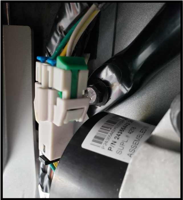
49. Secure the SRS connector to the cab harness using cable ties.
