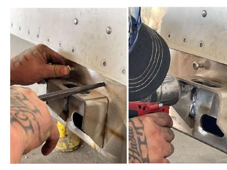
11. Using all existing holes as a guide, redrill all holes to their appropriate size. 5/16" thru the front of the floor, and 3/8" down both sides. Reinstall all fasteners and nut the floor screws.
