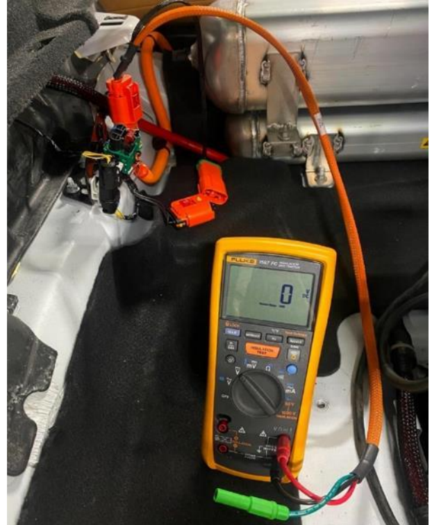
Figure 14 – PHEV Circuit Testing
