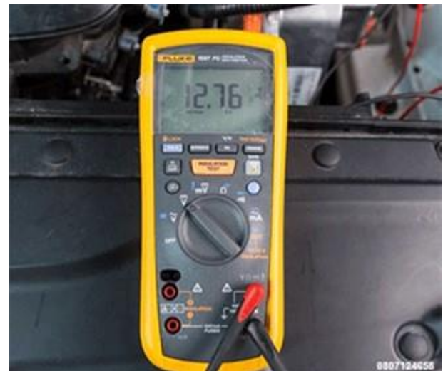
Figure 10 – PHEV Circuit Testing
