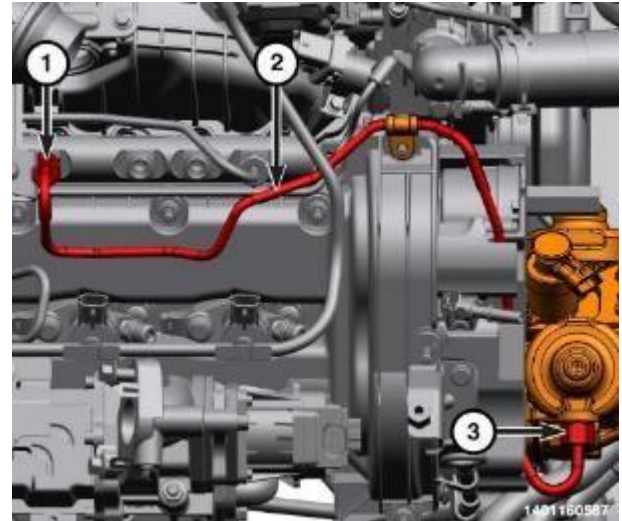
Figure 20 – Right Bank Fuel Supply
