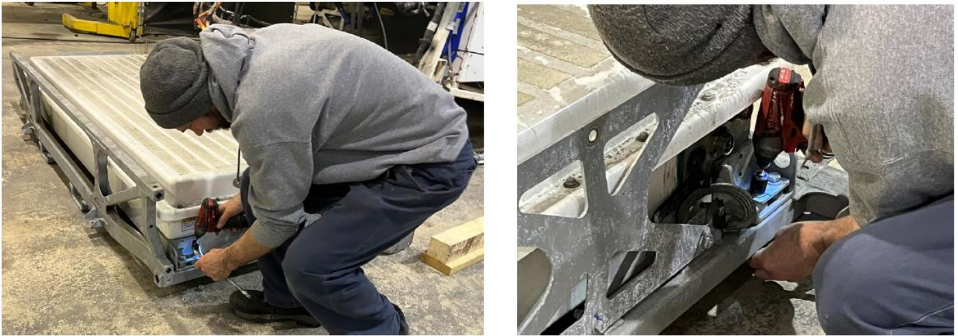
Figure 17: Removing Hardware from ESS Enclosure Feet
