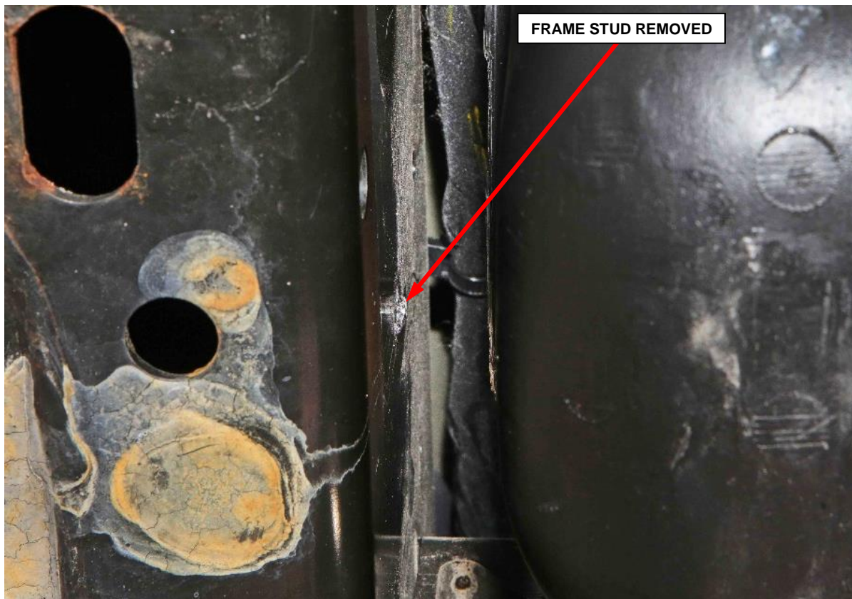
Figure 8 – Frame Stud Removed
