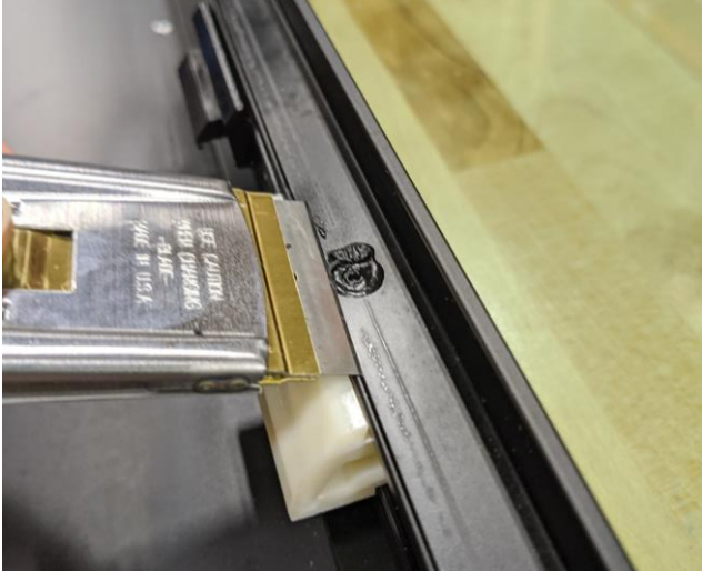
Figure 4a: Blade scraper removing sealant.
