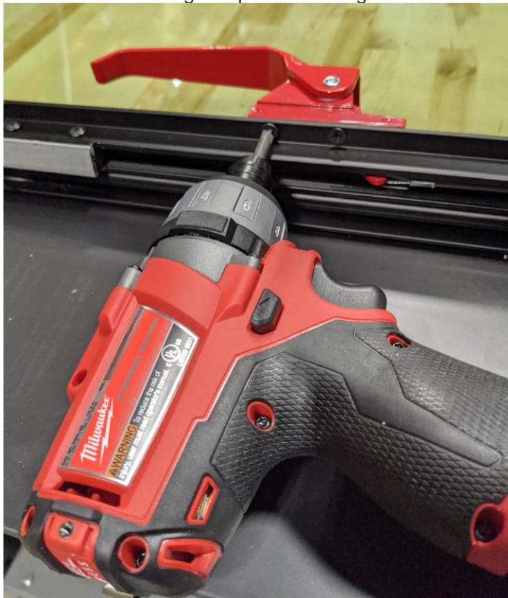
Figure 12: Removal of ER handle screws.
