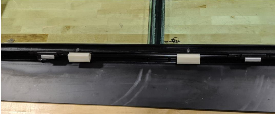
Figure 29: Locator blocks between ER latches.
