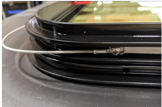
Figure 27b: Screw partially installed with ER cable loose.
