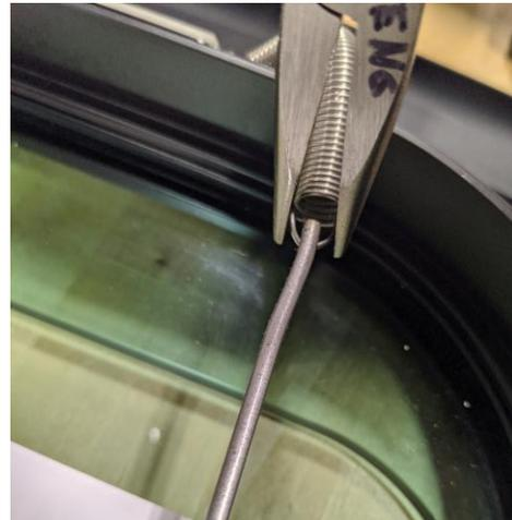
Figure 18b: Bend spring hook closed.
