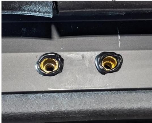
Figure 37: Sealant applied around rivet nut heads.
