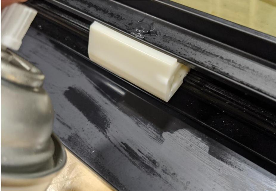
Figure 29: Silicone spray lubricant applied to locator block.
