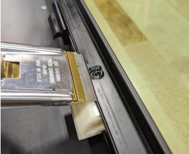
Figure 4a: Blade scraper removing sealant.
