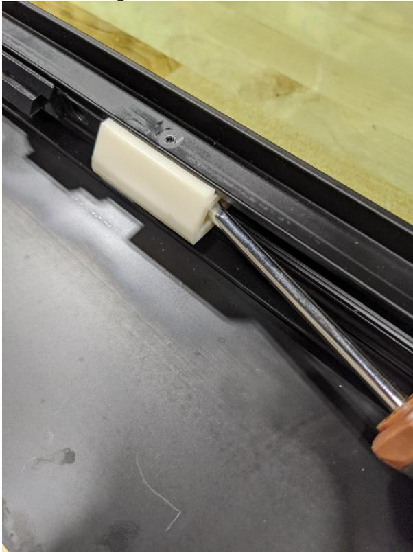
Figure 5a: Flat head screwdriver wedged in the side of the locator block.
