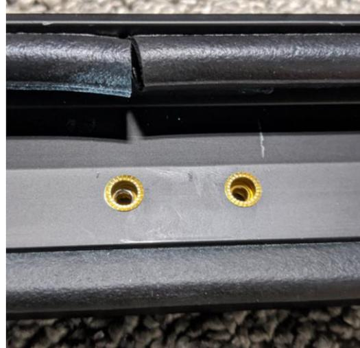
Figure 36b: Rivet nuts properly installed.
